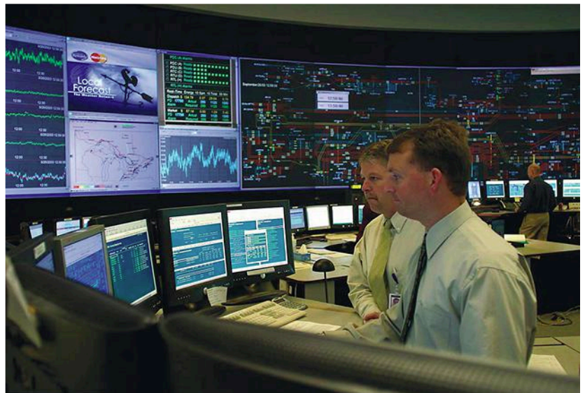
1. The control center of a large organization gets its raw data from sensors in the SCADA system. (Source: All About Circuits)
